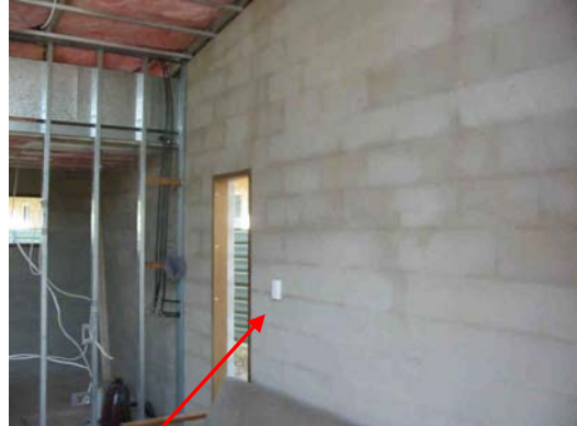
Inside west wall (4/05/06)
