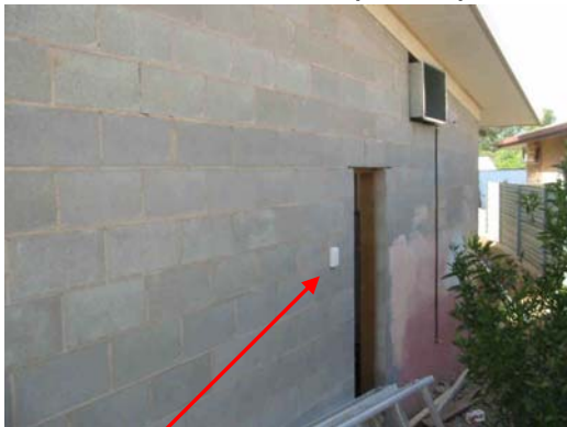
Outside west wall (4/03/05)
