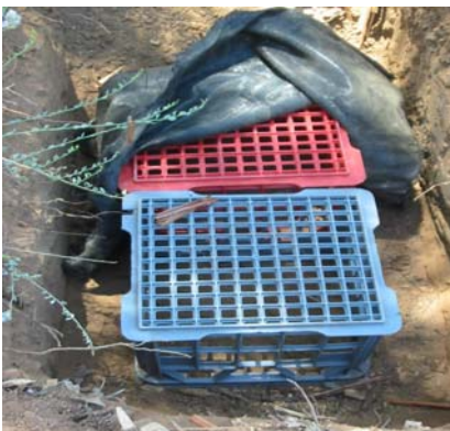
'Milk crate' subsurface tunnels covered by geotextile
